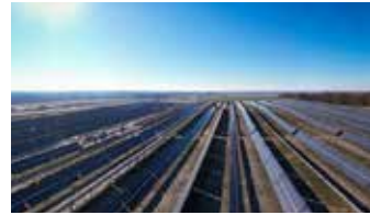
Dane County Airport Solar
