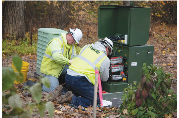
Crews install new facilities where overhead electric lines have been removed and replaced with underground lines as part of MGE's grid modernization projects.
