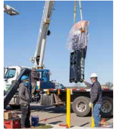
A large crane installed the fast charging station at the airport.
