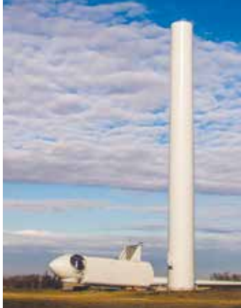
A rotor and nacelle rest next to one of Saratoga’s towers.
