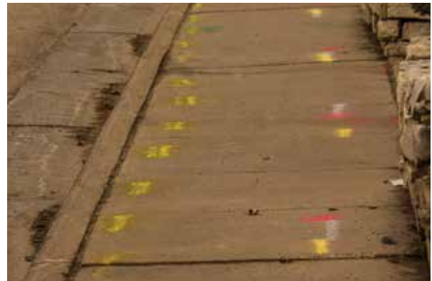
MGE is using a more environmentally friendly paint option for marking buried utility lines.
