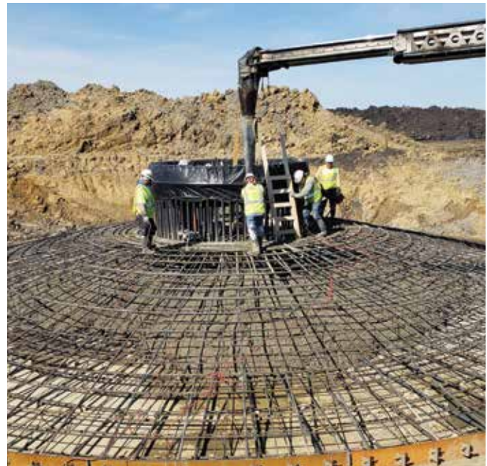
Crews prepare a foundation for one of 33 turbines at MGE's Saratoga wind farm.
