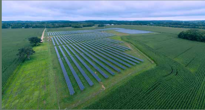
Left: MGE's 6-megawatt Tyto Solar project came online in early 2024. A distributed energy resource, the facility feeds carbon-free energy directly to MGE's distribution grid serving customers. During the growing season, sheep from a nearby farm graze at the facility to keep the grasses and brush from shading the panels.
