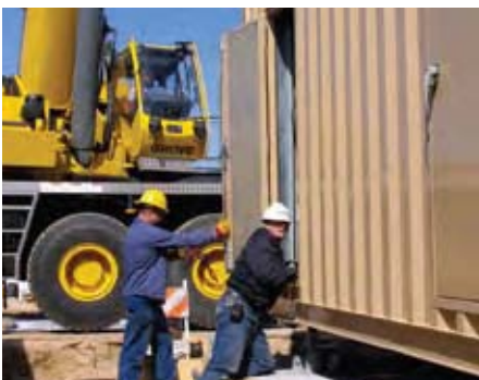
Crews guide one of MGE's backup electric generators into place at the new TEAM Technologies data center.
